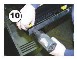
10. Tighten all 4 bolts and torque to 85 ft. lbs.
